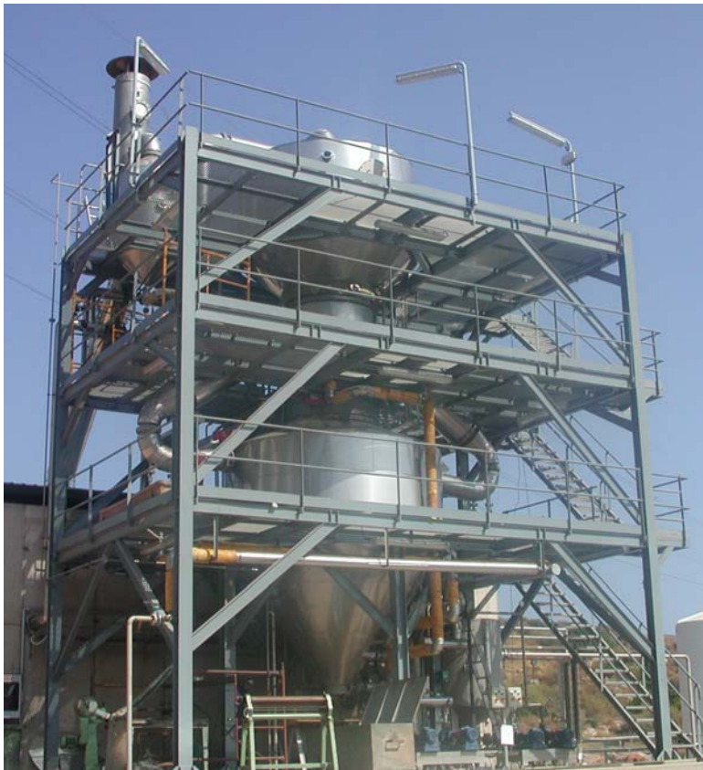
ZLD for landfill leachates
